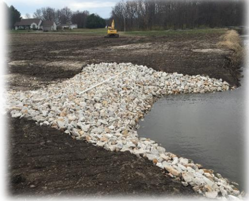
Grade Control Structure
