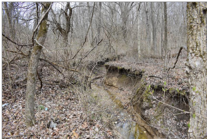
Eroding Forested Gully
