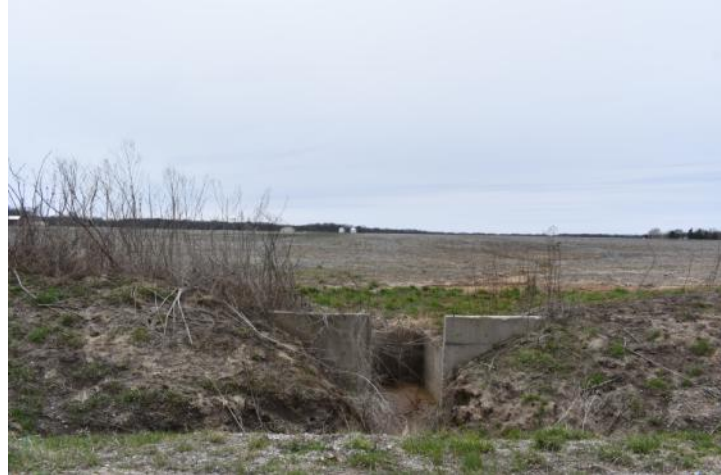
Erosion Control Structure
